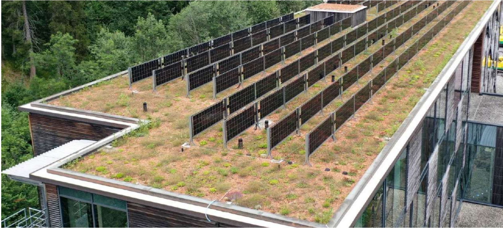
Photo Courtesy of ZinCo GmbH
