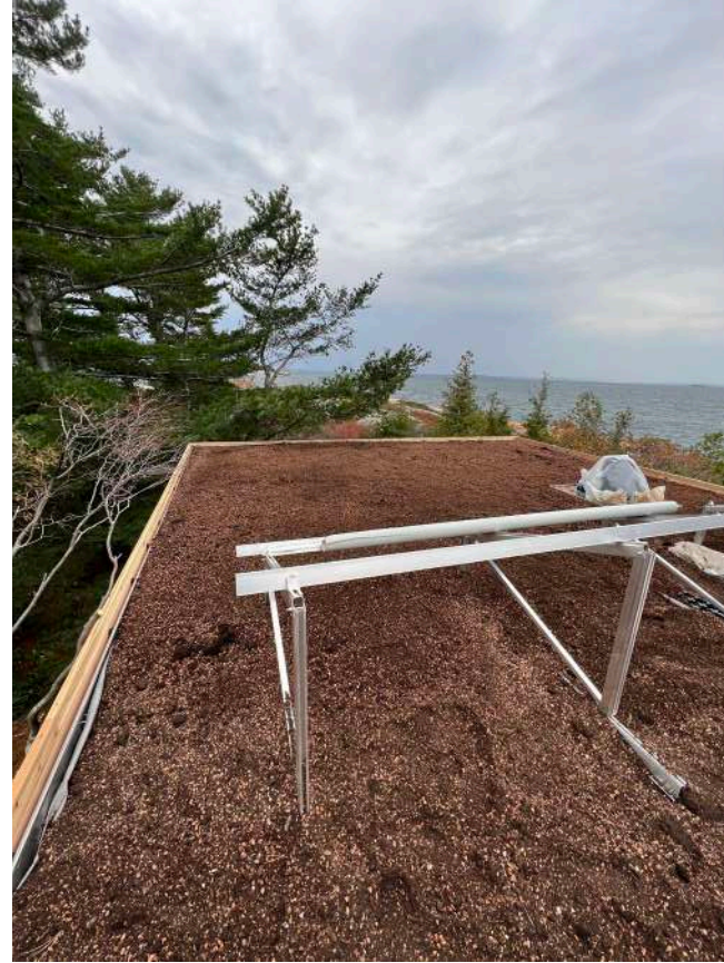
FLL Substrate – Necessary for Uplift
