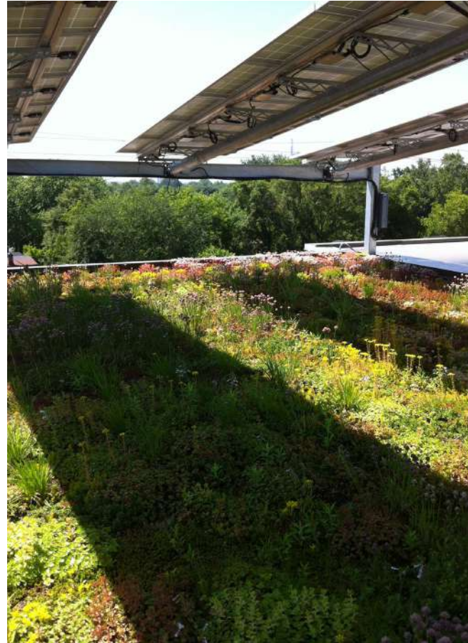
Riverdale Hub Toronto, arguably first green roof and PV in Canada that integrated Agriculture
